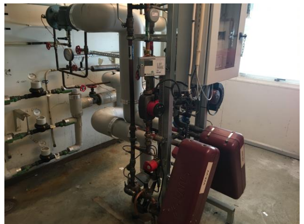
Undercentral, tryckstyrd VVC-pump.
